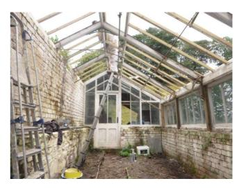
Renovation has now been started on the remaining section to complete the project. The glass in the roof has been removed, repairs are being undertaken to replace the door glass and broken panes. We hope to have it painted and roofed by the autumn term. As far as possible we have retained the original features including the ironmongery and the tiled floor.
